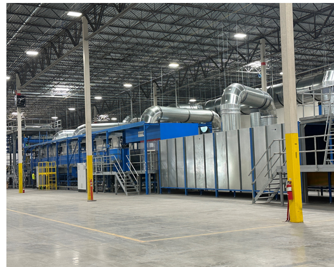
The pouring line inside the facility.
