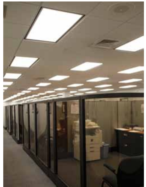
Lighting Retrofits - Most Leggett facilities use high-efficiency lighting systems that reduce energy consumption by almost 50% and create a brighter, safer work environment.
